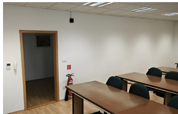
Fig. 2 IAQ unit in classroom
